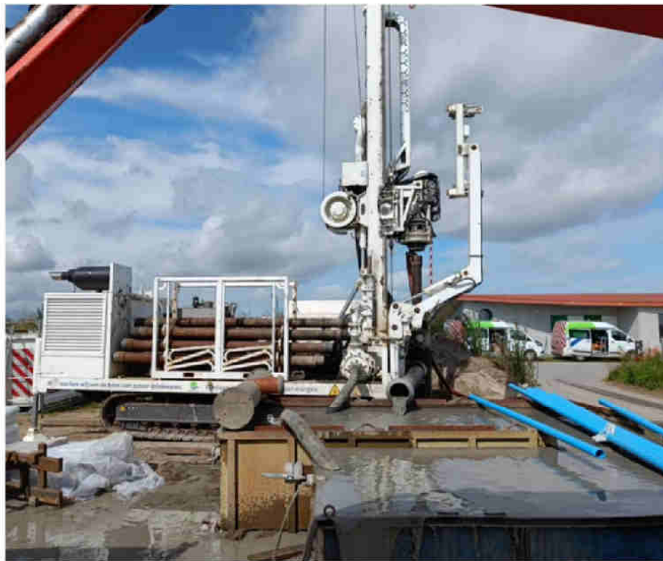
Figure 3.5: Drilling of monitoring well PB6o/d.
