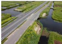
<Faunapassage langs de N210 in de Krimpenerwaard.>
