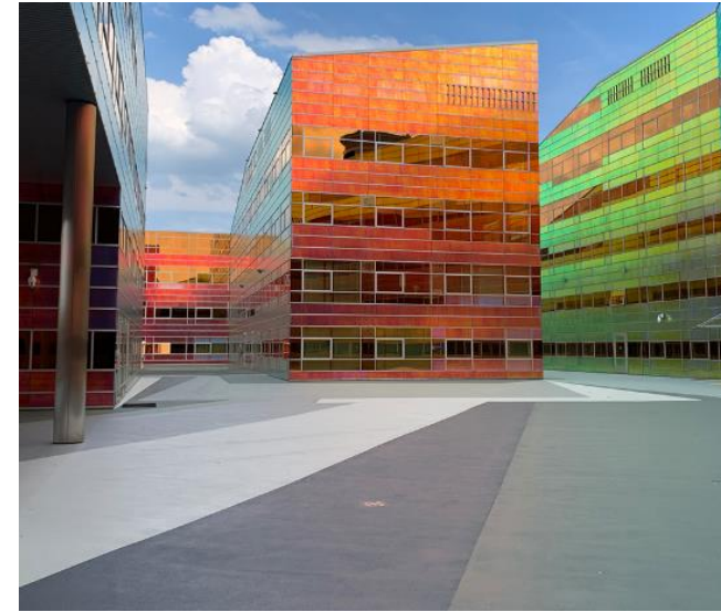
Epoxy vloercoating Metex / Triflex
