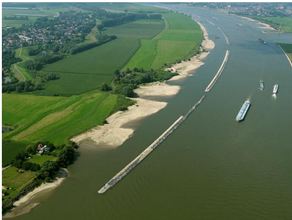
Figure 19 - Construction of longitudinal dams in the Waal can significantly reduce the hydraulic turbulence in the shore zone.
