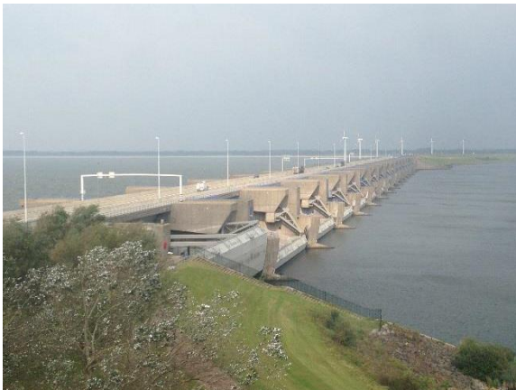
Figure 14 – Haringvliet sluices, the storm surge barrier between the mouth of the Rhine and the North Sea.
