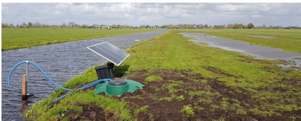
Foto: Waterinfiltratiesysteem (WIS)
