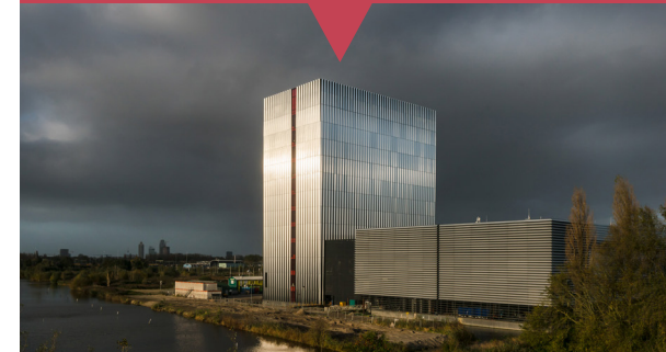
Datacenter Equinix AM3
