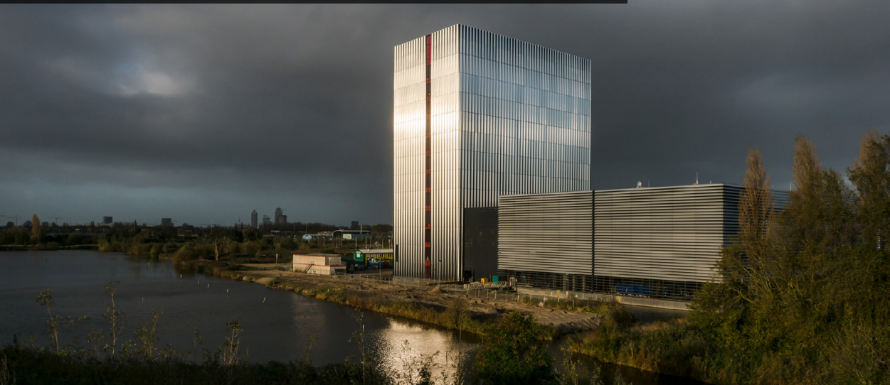
Datacenter AM3 en AM4 in Amsterdam
